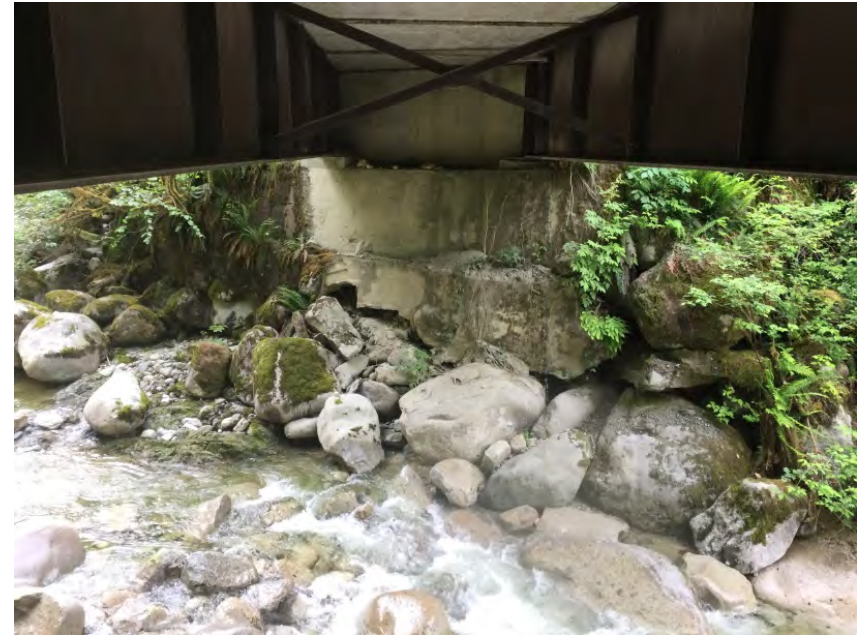
Left Bank Abutment when facing downstream
