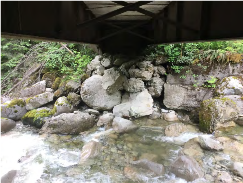
Right Bank Abutment when facing downstream
